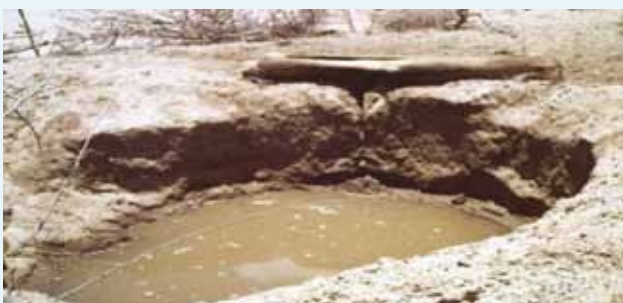
Shallow dug well on a river bed
