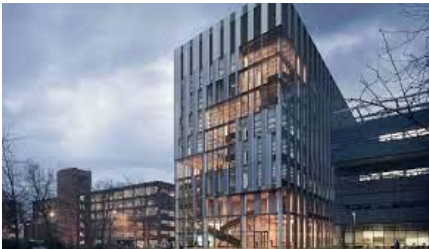
Royce Hub Building, University of Manchester
